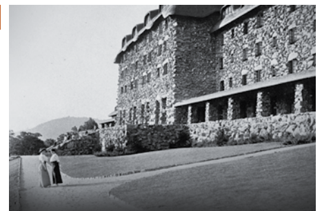
› The original portion of the Grove Park Inn (above) was built of granite boulders dug out of the mountain. The course layout dates to 1899.
